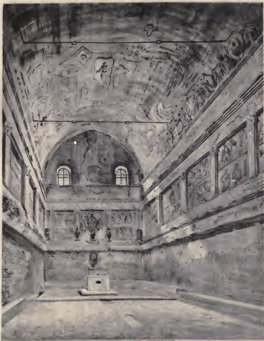
VIEW OF THE INTERIOR
